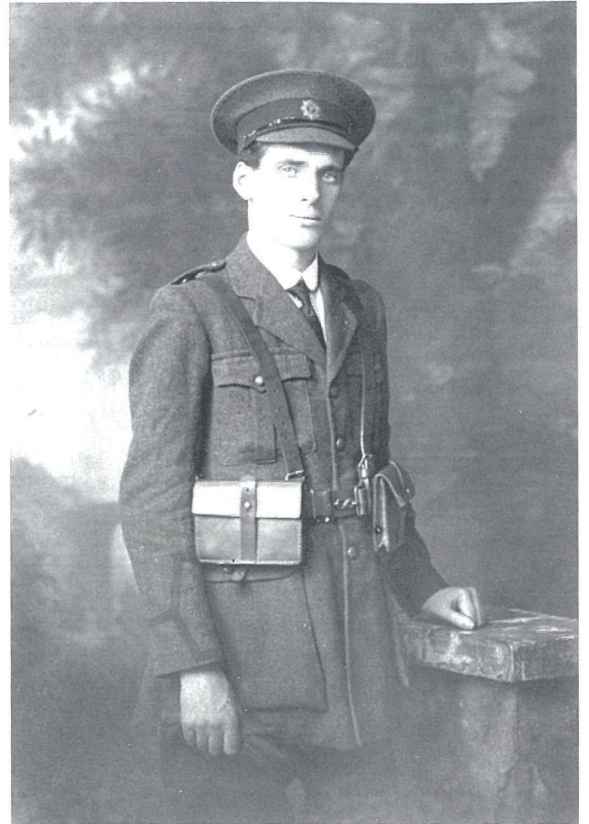
Michael Staines Photo courtesy of Garda Museum, Dublin.
